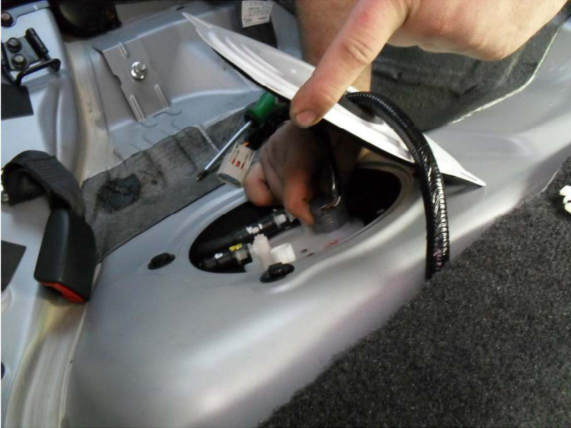
4. Cover the plastic fuel lines with a rag, press the lock tabs, and remove the fuel lines from the bulk head.
